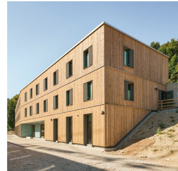
Close to the biological cycle: the straw-bale building of Plankstetten Abbey, House St. Wunibald
