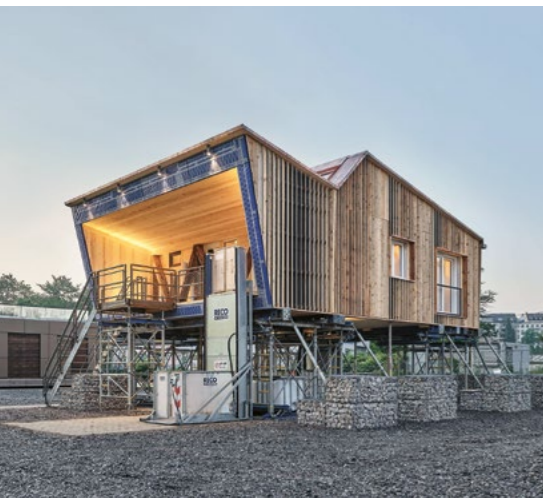
The recyclable RoofKIT prototype for renovations and building additions in urban development
