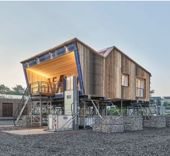
The recyclable RoofKIT prototype for renovations and building additions in urban development
