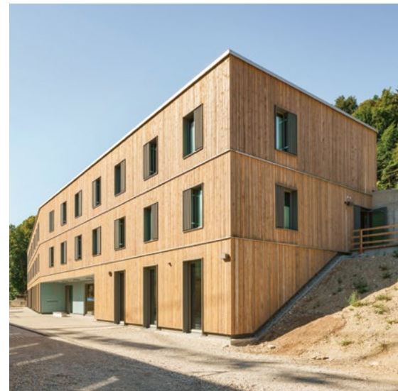
Close to the biological cycle: the straw-bale building of Plankstetten Abbey, House St. Wunibald
