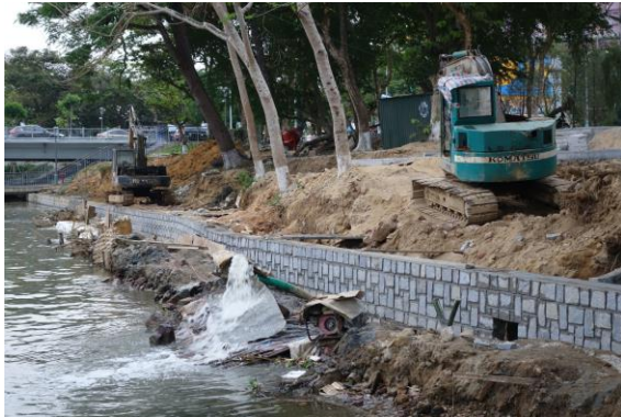
Figure 14: Construction site in Hue (@dena / Moritz Limbacher)
