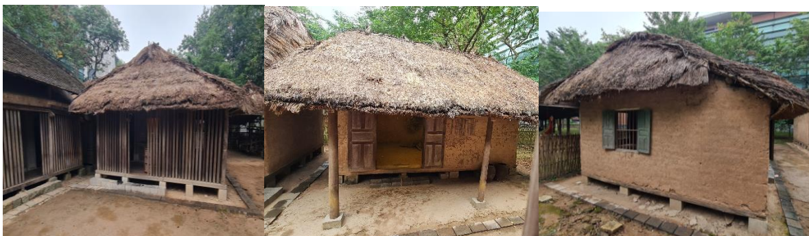
Figure 6: Examples of vernacular houses (©dena / Stefan Schirmer)
