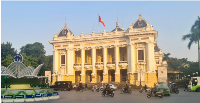
Figure 9: The Hanoi Opera House built by the French colonial administration between 1901 and 1911 (@dena / Stefan Schirmer)
