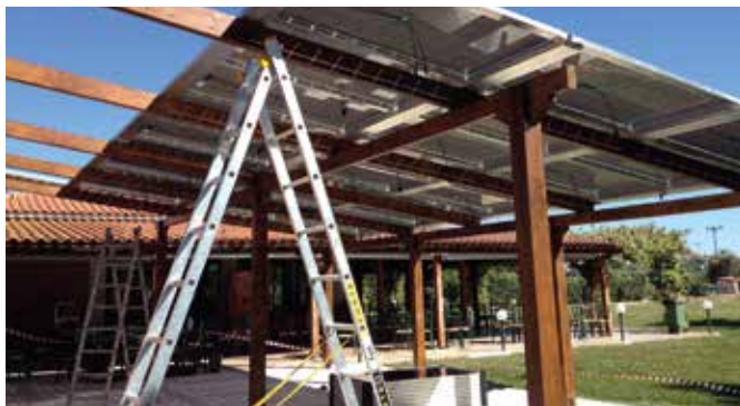
Montage der Anlage – Installation of the system
